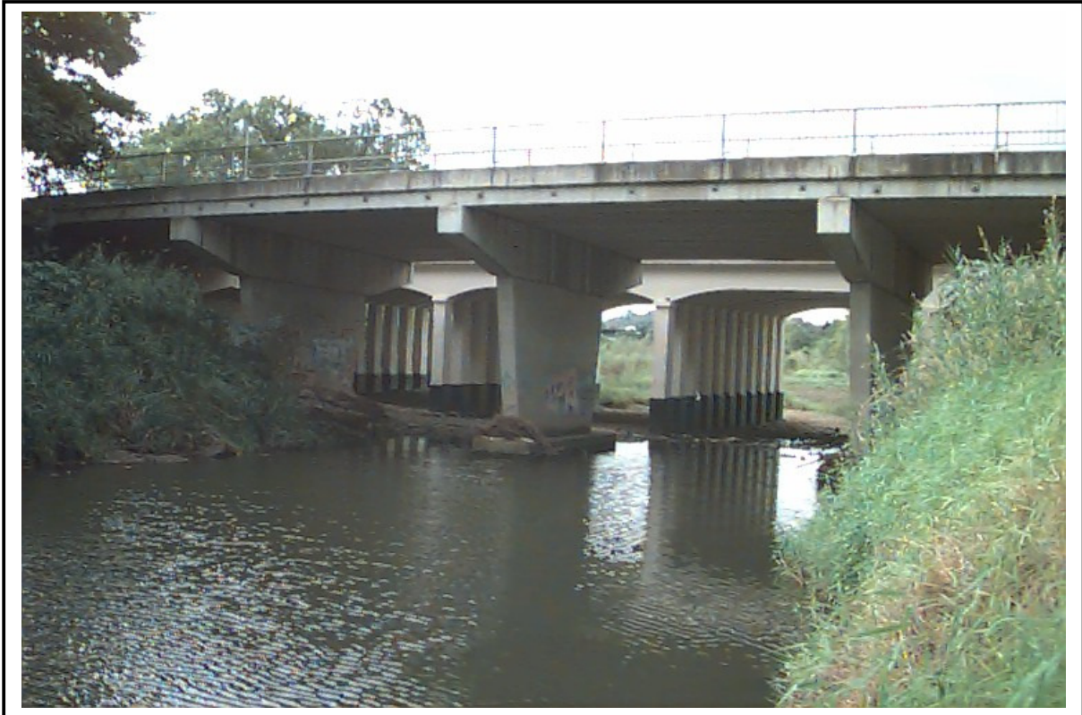
Kelvin Grove Road (Outbound), looking downstream
