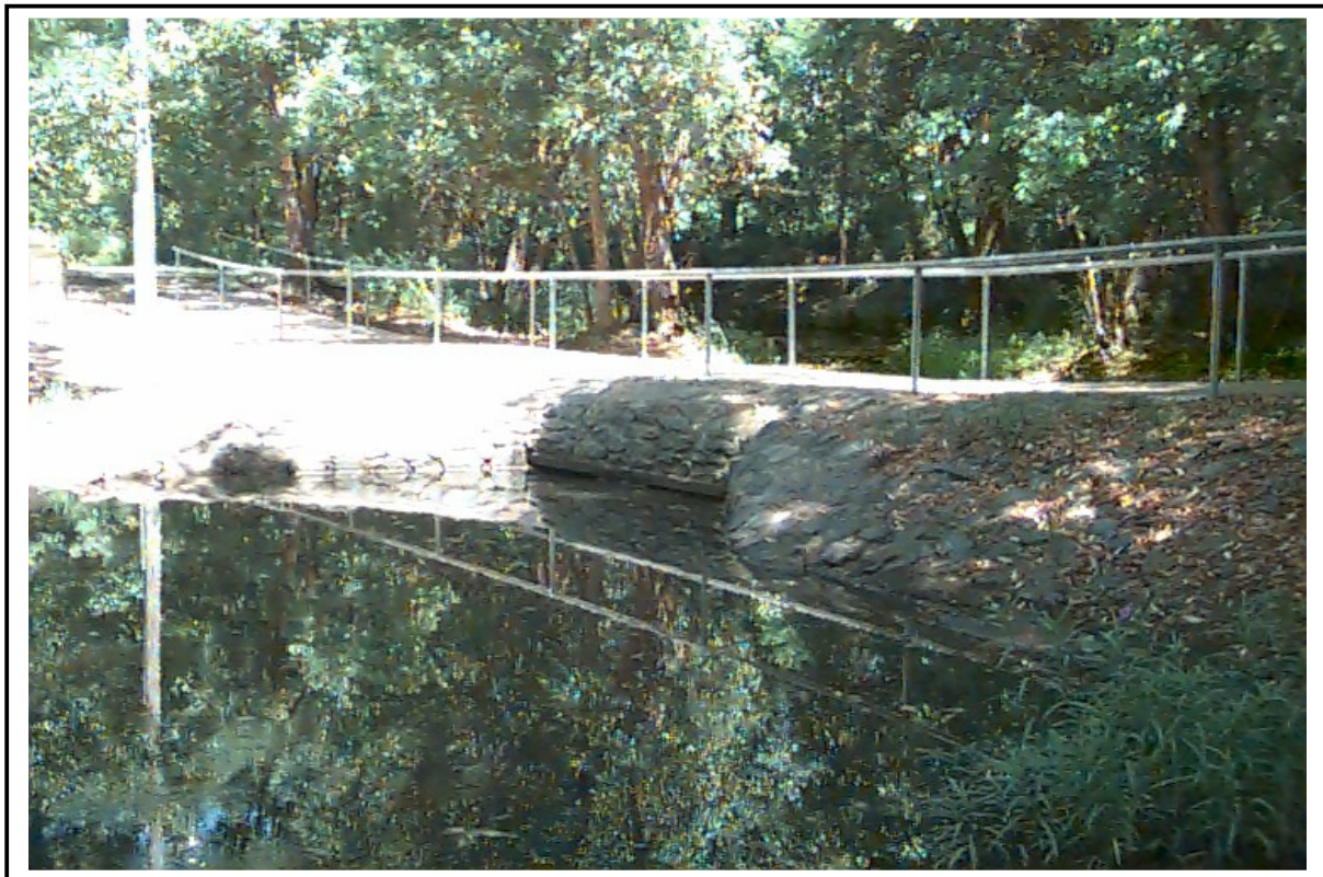
Tandara Street Footbridge, looking upstream
