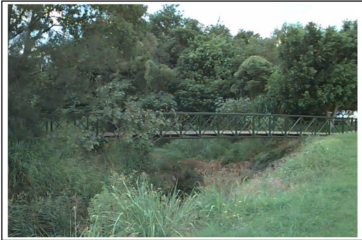
Nathan Avenue Footbridge, looking upstream
