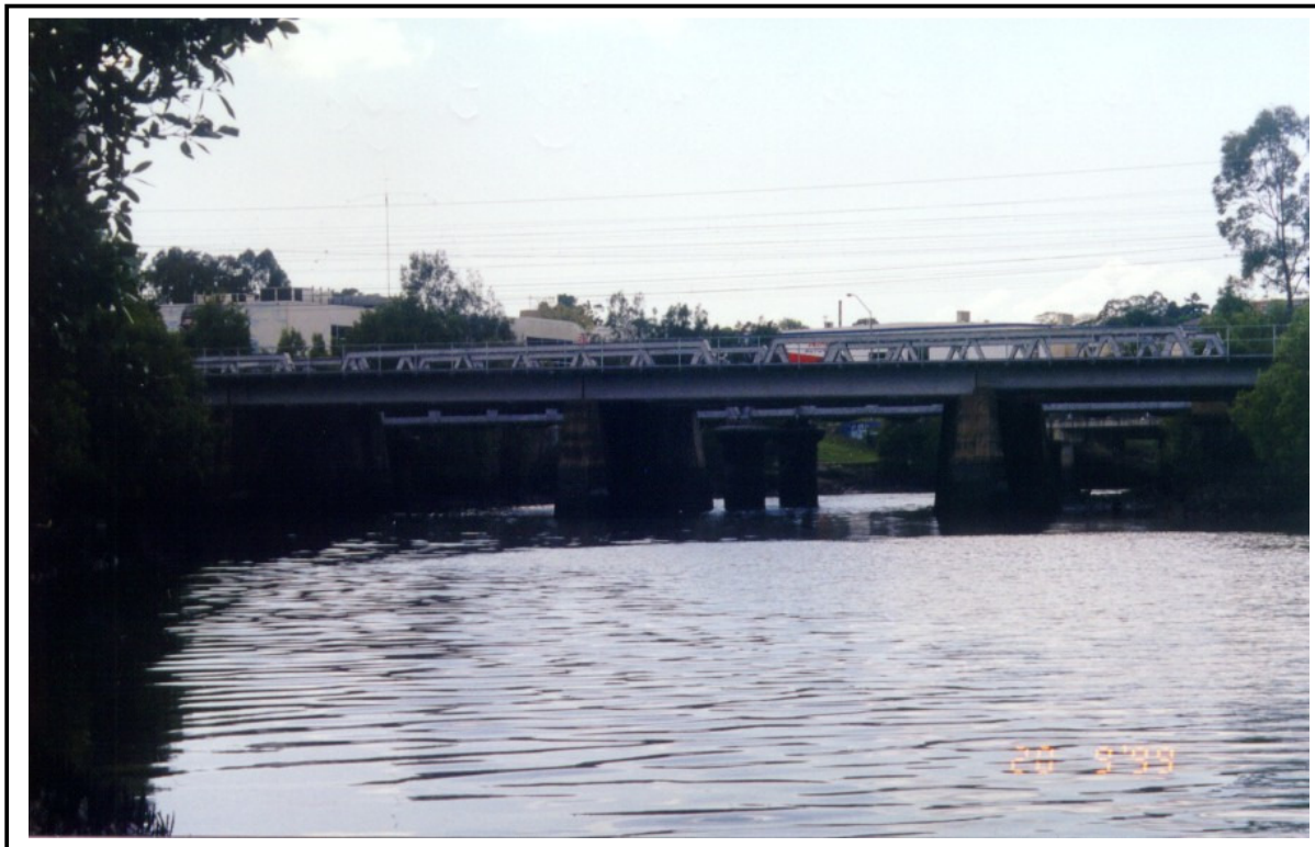
North Coast Railway, looking downstream
