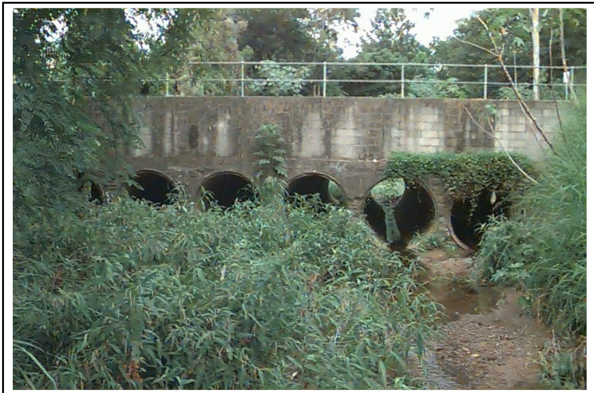
Settlement Road, looking upstream
