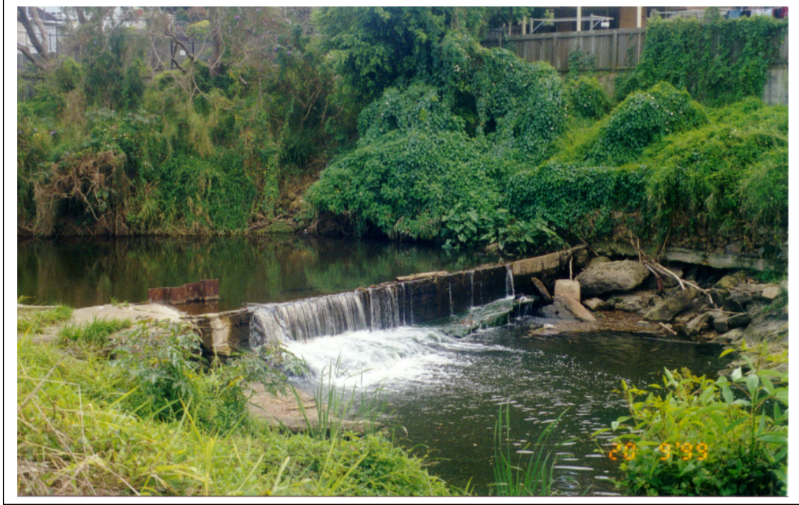
Figure A.11 Bancroft Park Gauge Rating Weir
