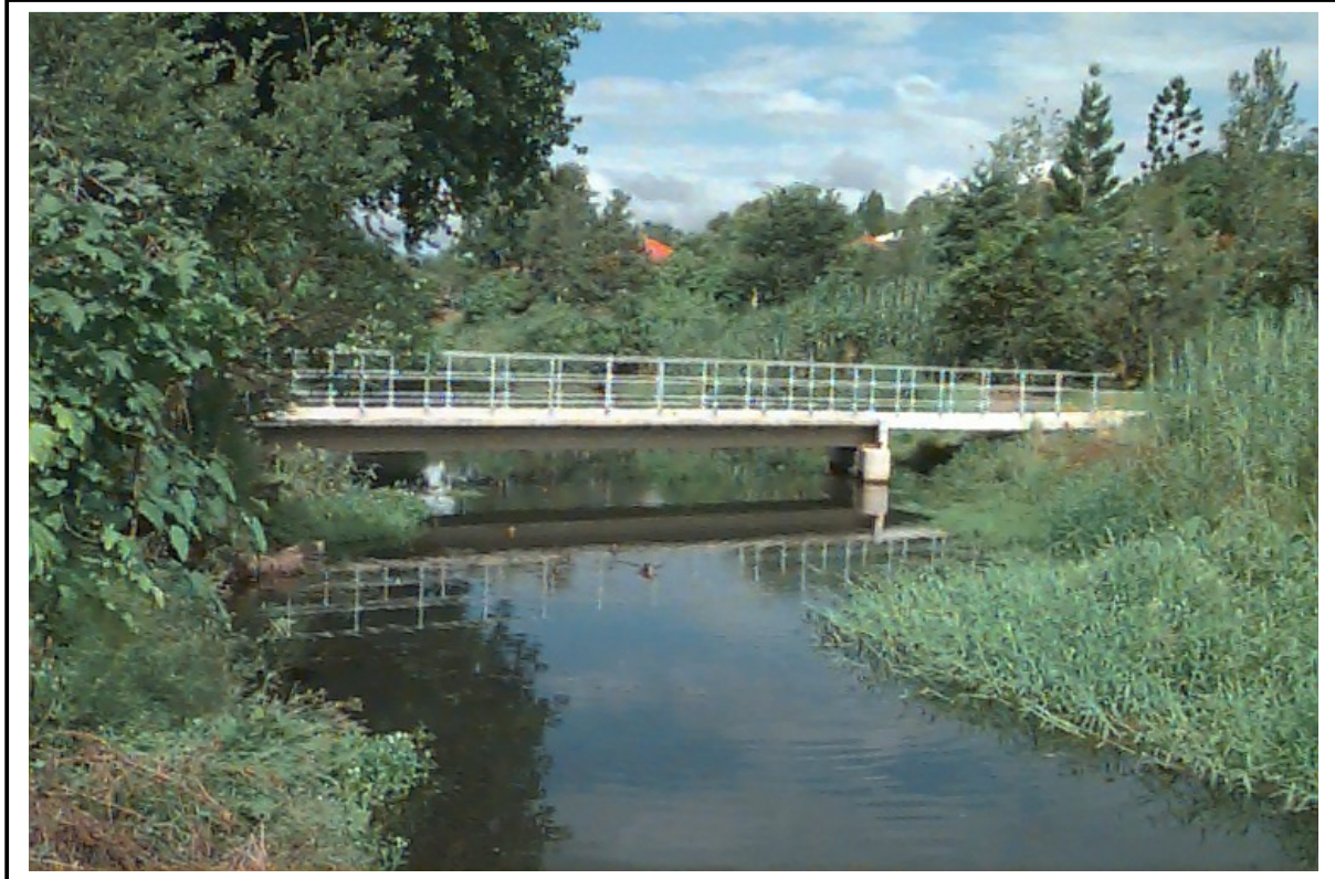
Murray Street Footbridge, looking downstream
