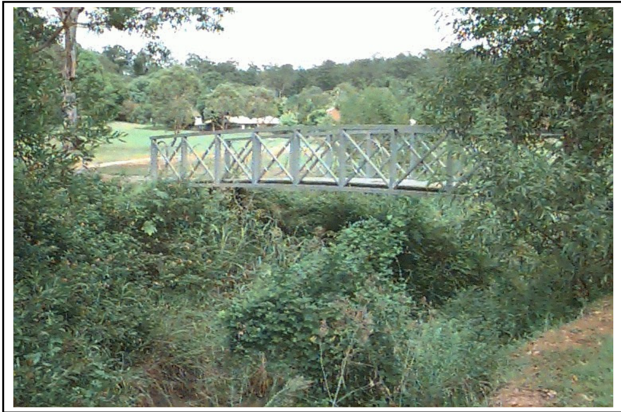
Wittonga Park Footbridge, looking upstream
