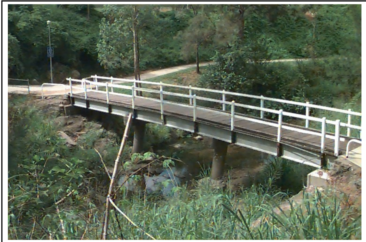
Royal Parade Footbridge, looking upstream
