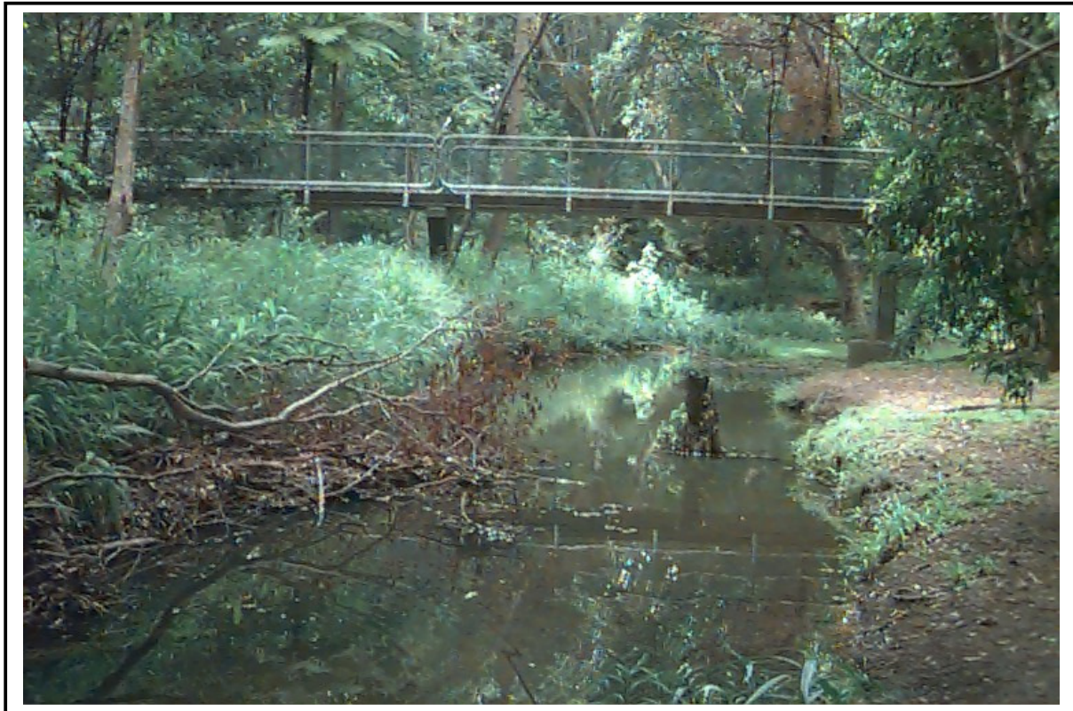
Lilley Avenue Footbridge, looking downstream
