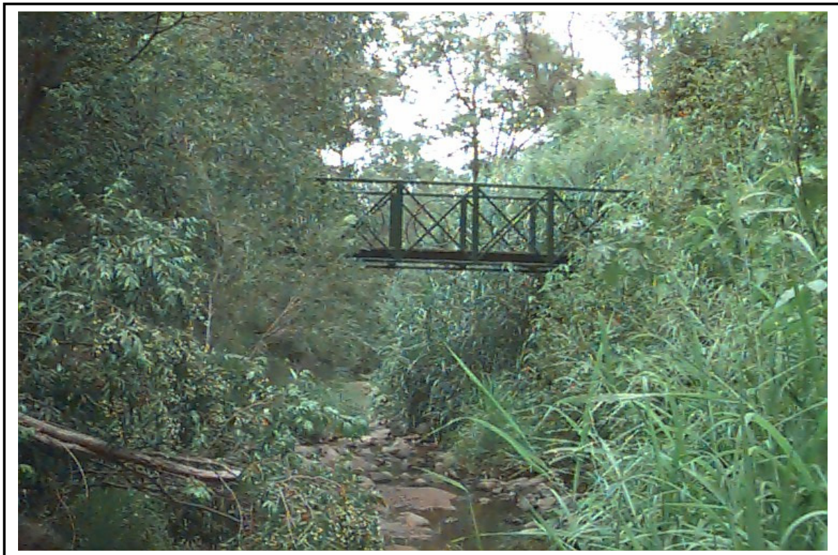
Lochinvar Lane Footbridge, looking downstream
