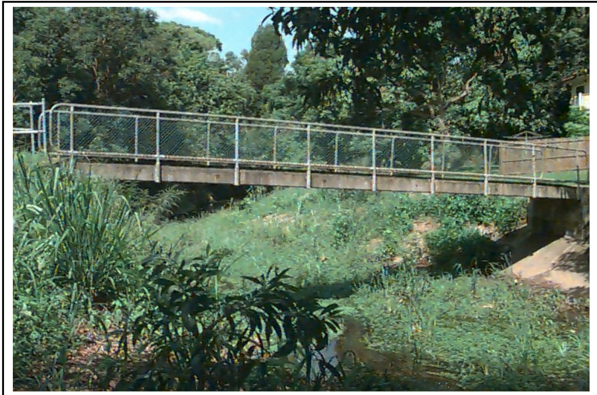
Devonshire Street Footbridge, looking downstream
