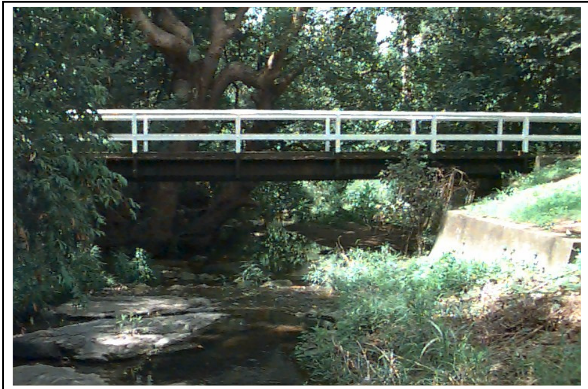
Coolibah Street Footbridge, looking downstream
