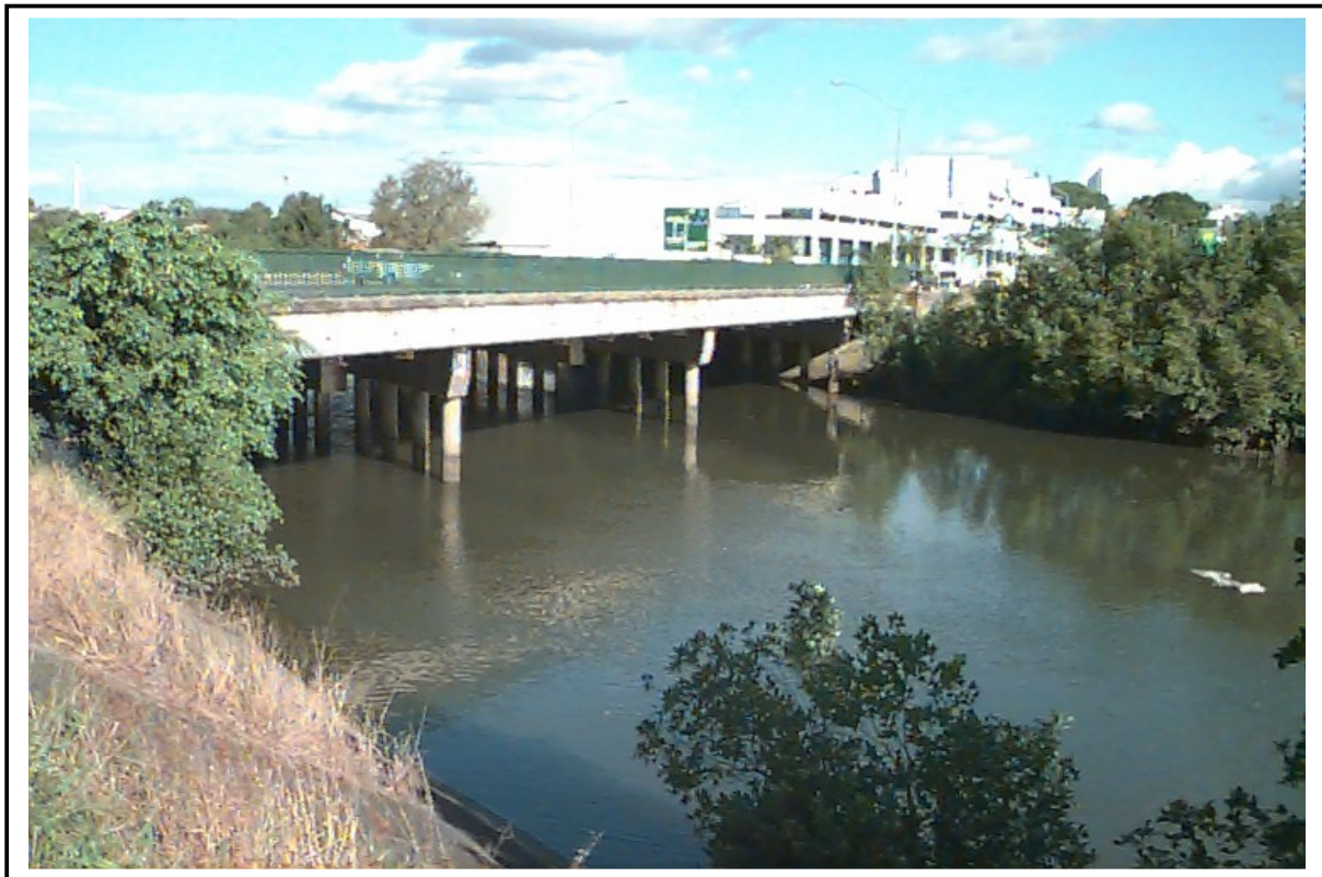
Bowen Bridge Road, looking downstream
