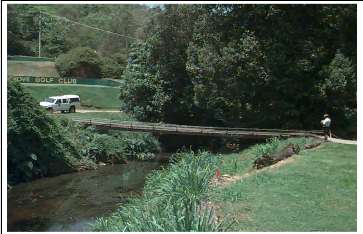
Ashgrove Golf Course Footbridge No 2, looking downstream
