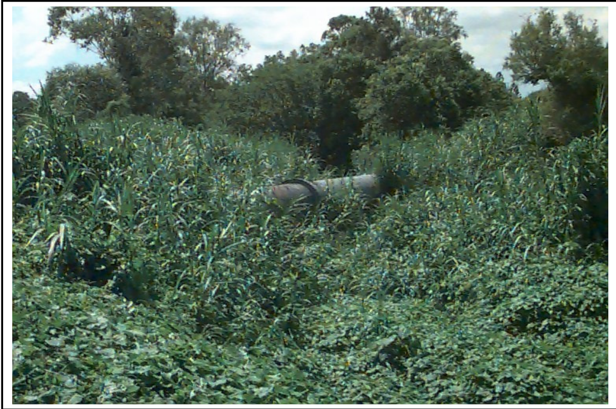
Kamber Street Pipe, looking downstream
