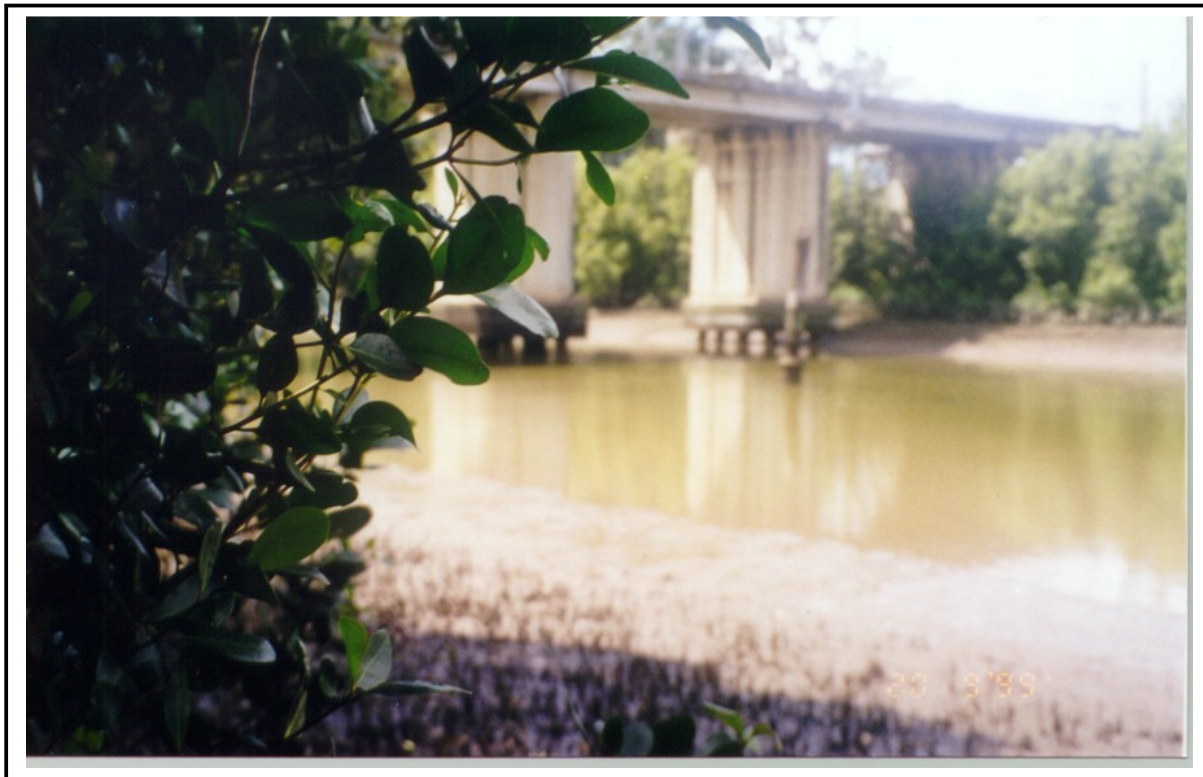
Ferny Grove Railway, looking downstream
