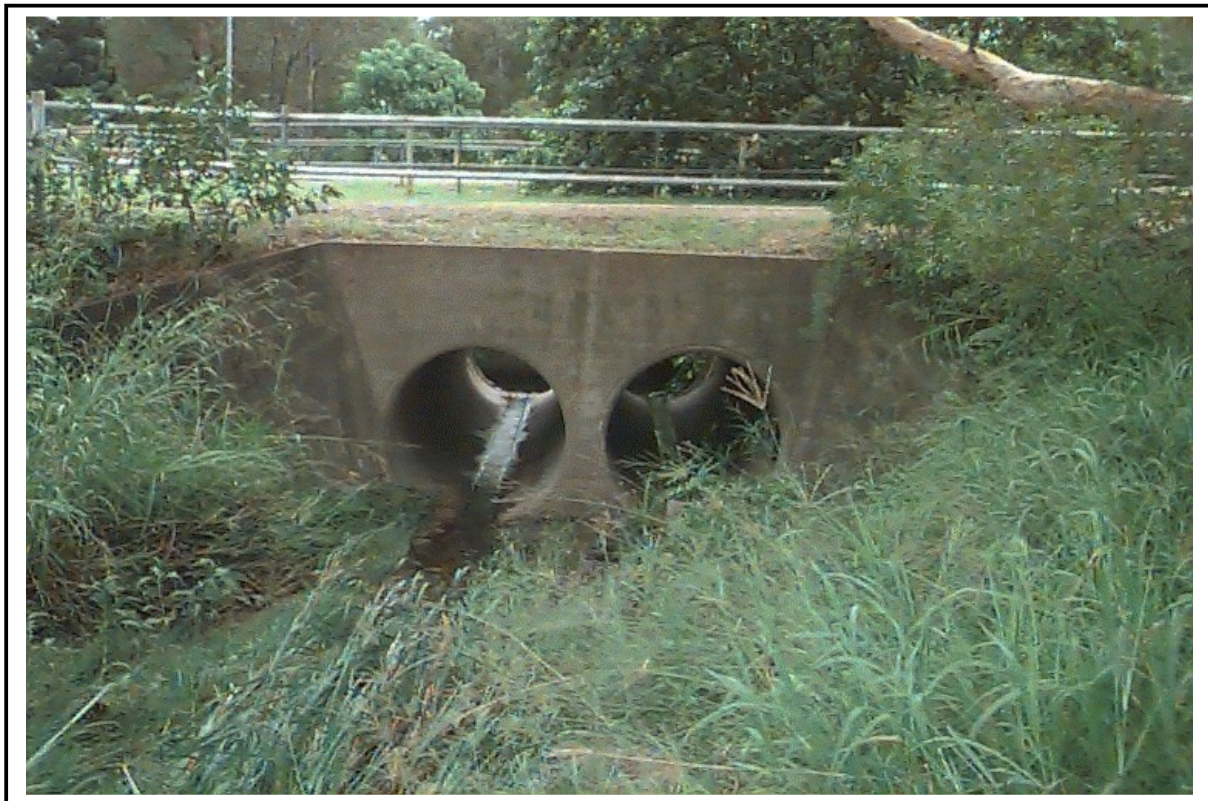
Wittonga Park Footpath, looking downstream
