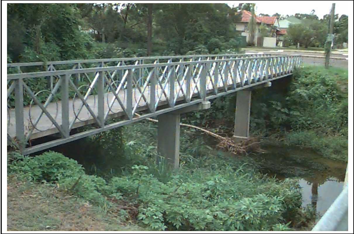
Mirrabooka Road Footbridge, looking upstream
