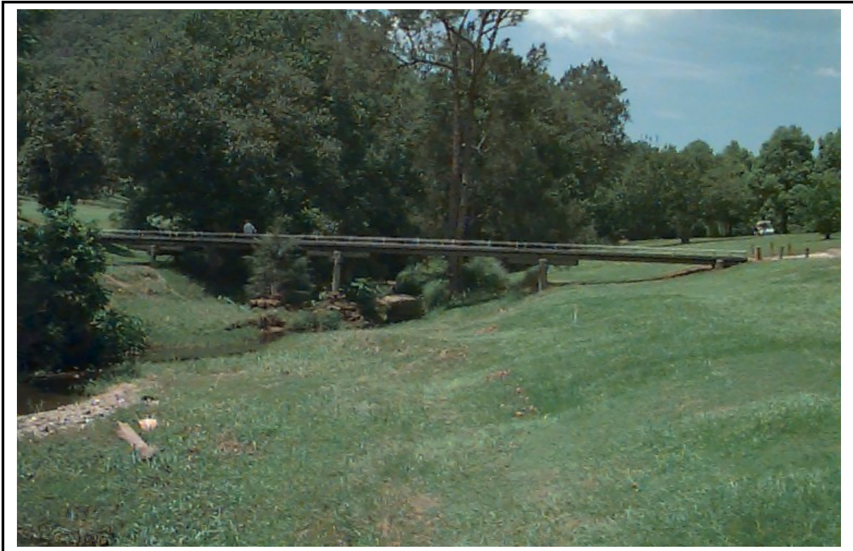
Ashgrove Golf Course Footbridge No 3, looking downstream
