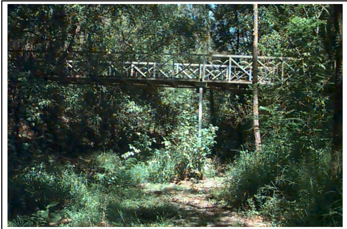
Riaweena Street Footbridge, looking downstream
