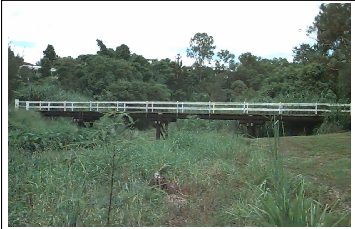
Steege Street Footbridge, looking downstream
