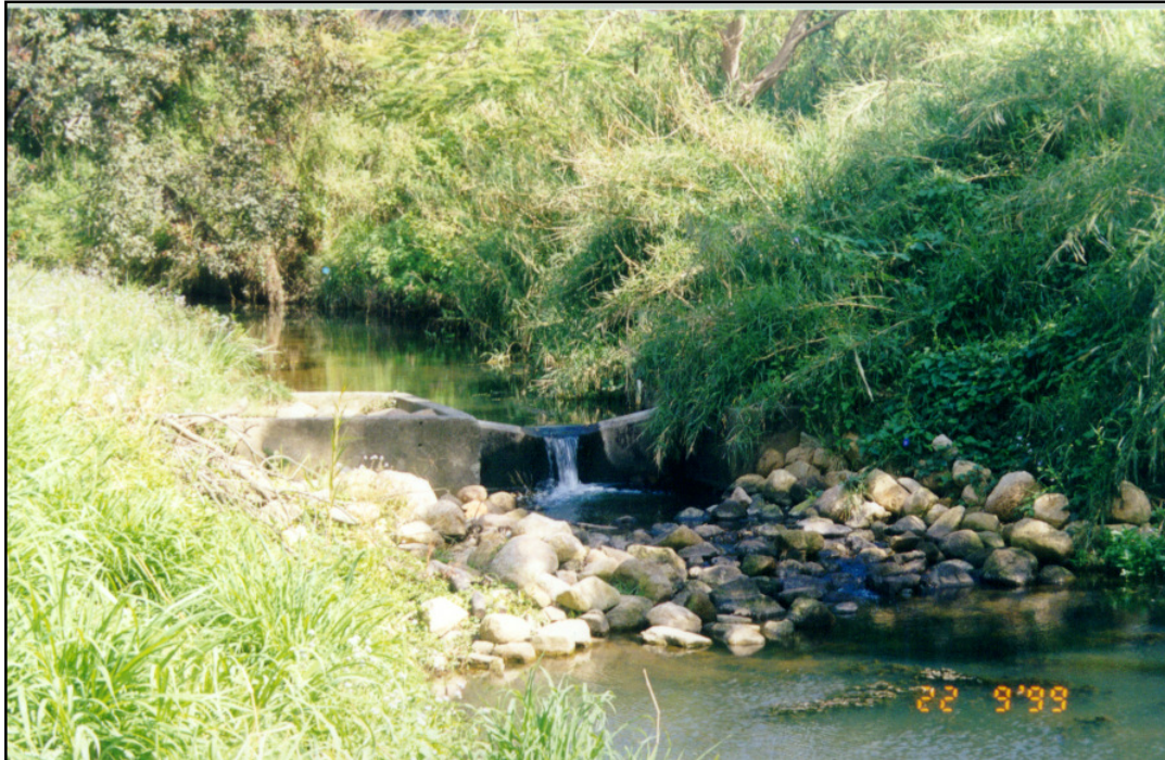
Figure 4.5 Jason Street Rating Weir
