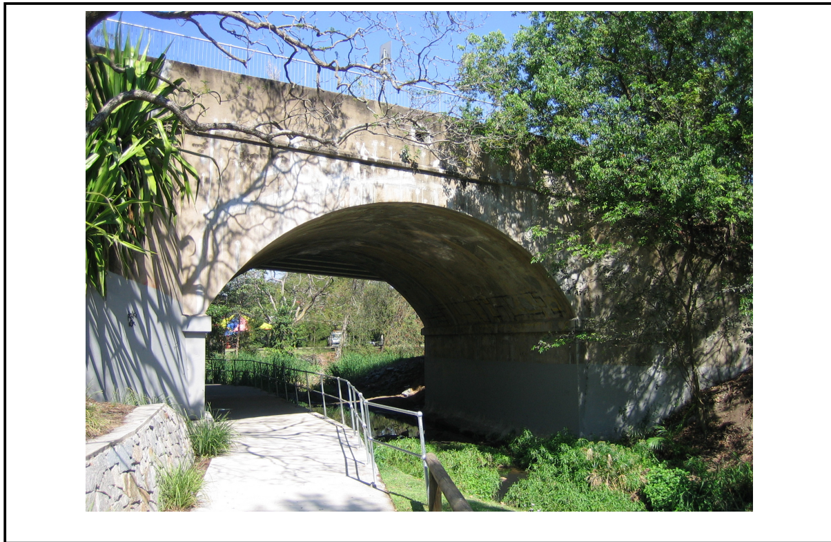
Waterworks Road, looking upstream
