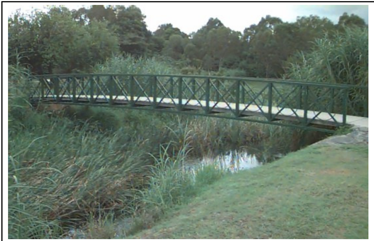
Corbie Street Footbridge, looking downstream
