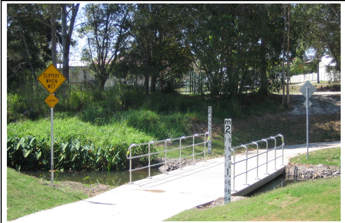
Quondong Street Bikeway bridge
