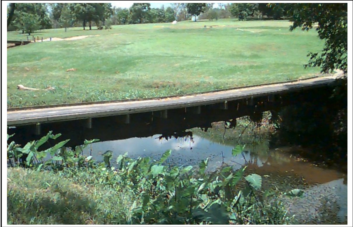
Ashgrove Golf Course Footbridge No 4, looking downstream
