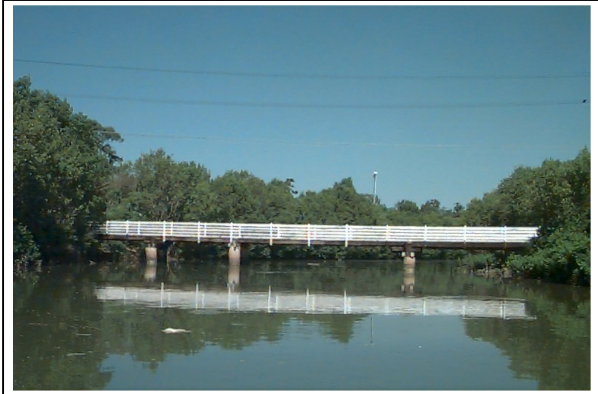
Bishop Street Footbridge, looking downstream
