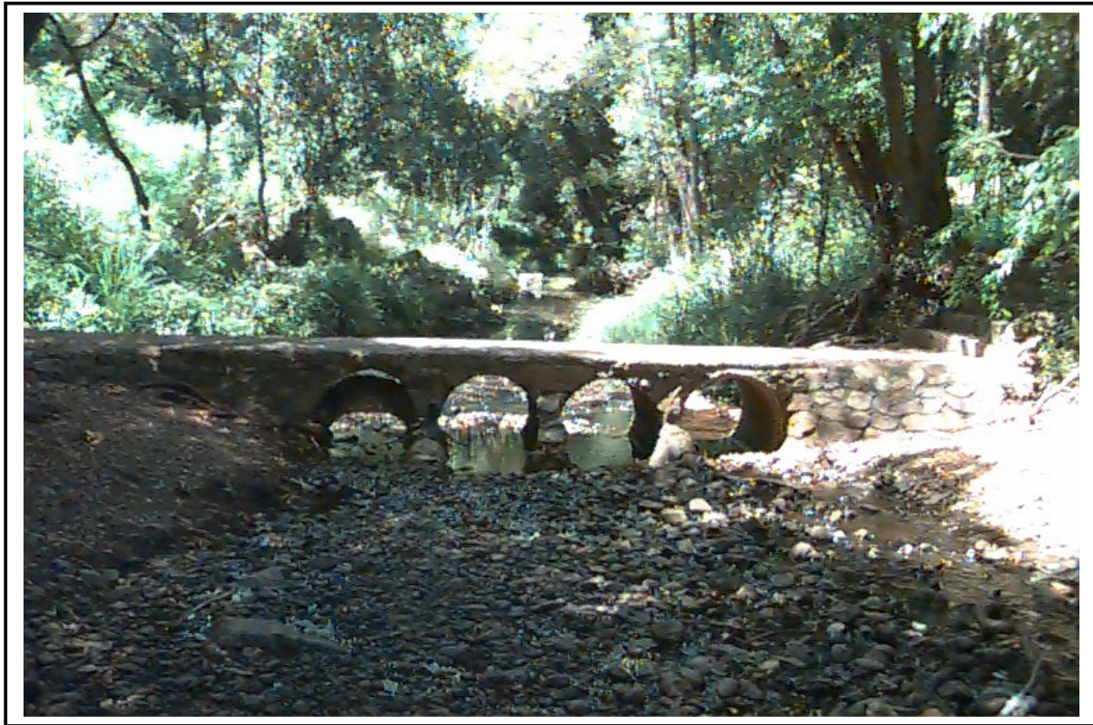
Walton Bridge Causeway, looking downstream
