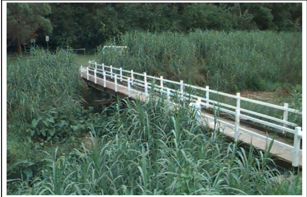
Park Avenue Footbridge, looking downstream
