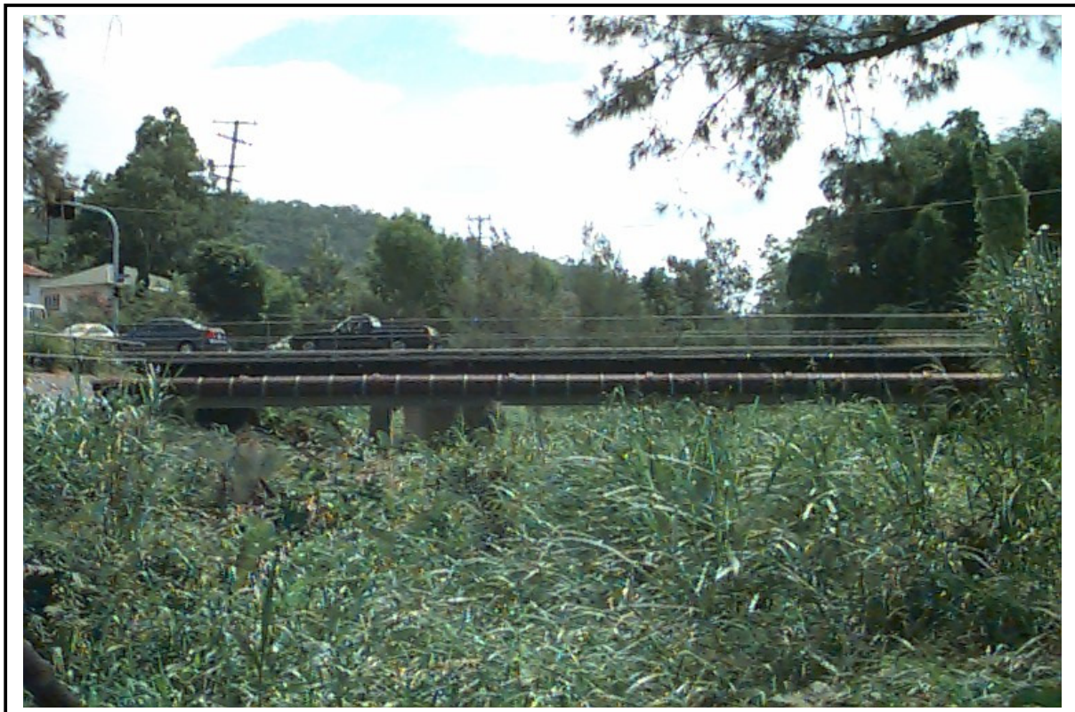
Gresham Street, looking upstream
