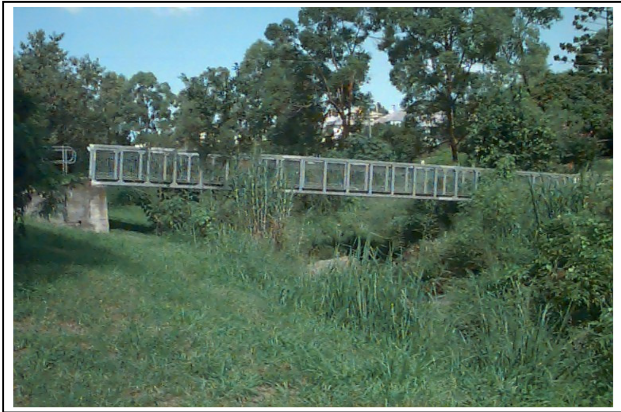
Lugg Street Footbridge, looking downstream
