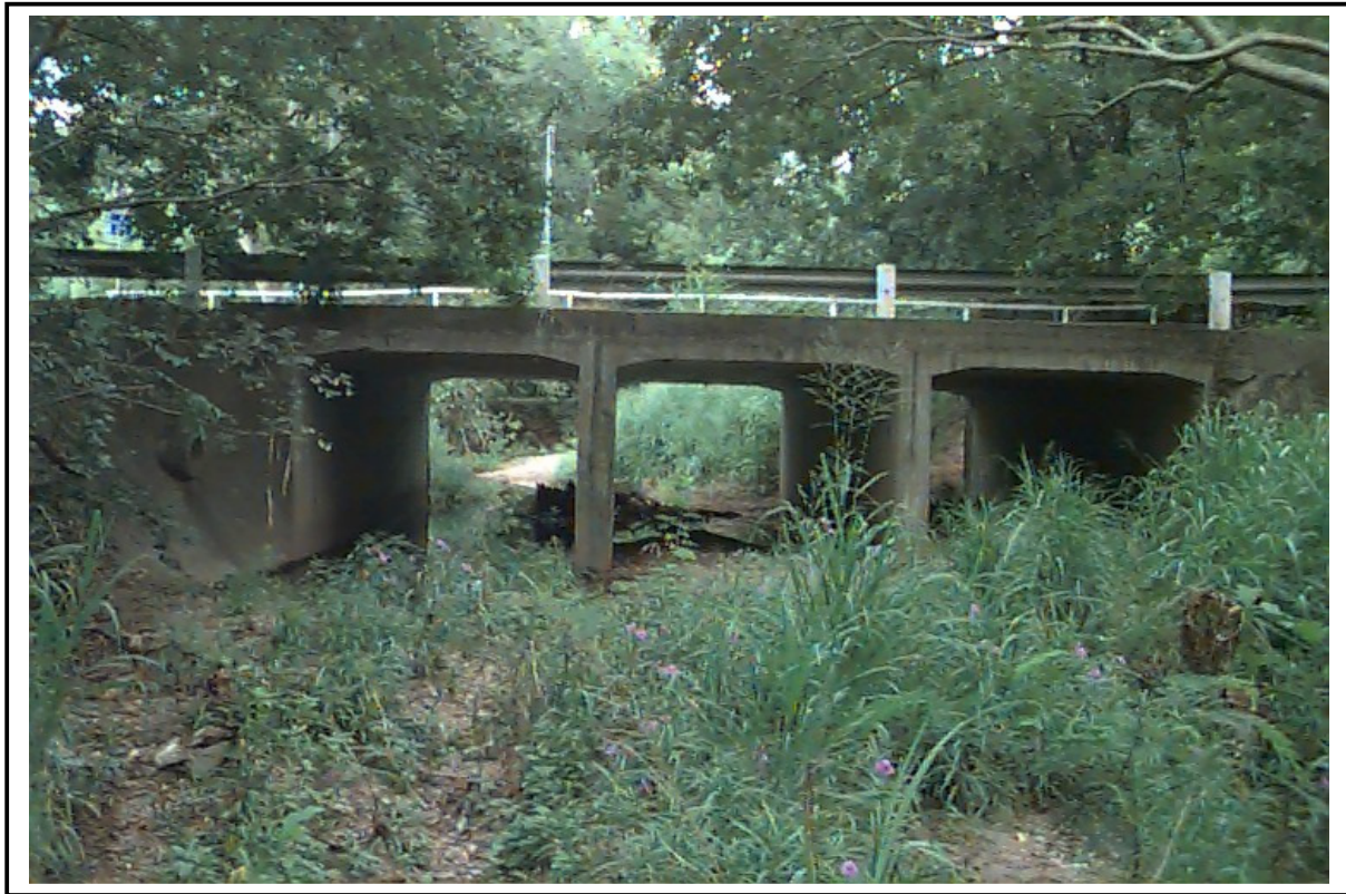
Glenrosa Road, looking downstream
