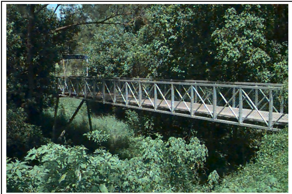
Shopping Centre Footbridge, looking upstream
