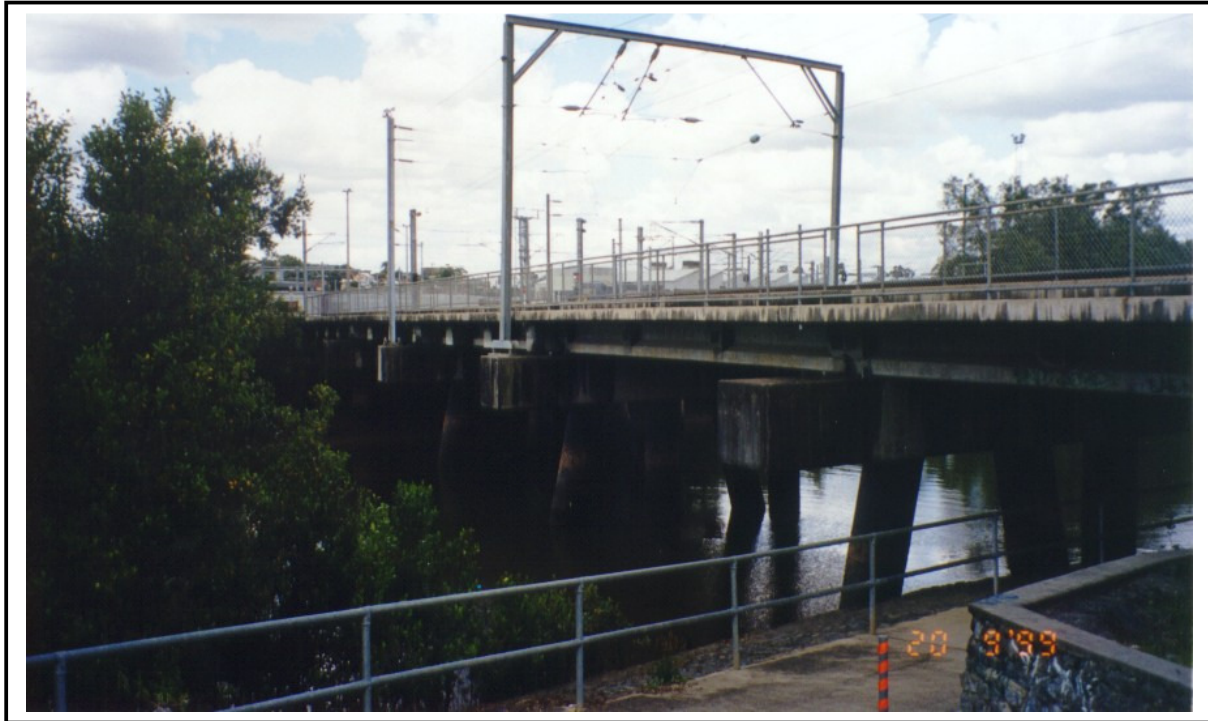
Railway Loop, looking downstream
