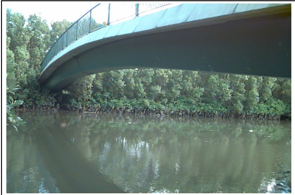
Downey Park Footbridge, looking upstream
