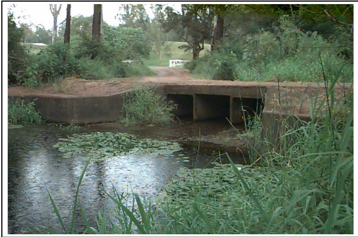
Dam Causeway, looking upstream
