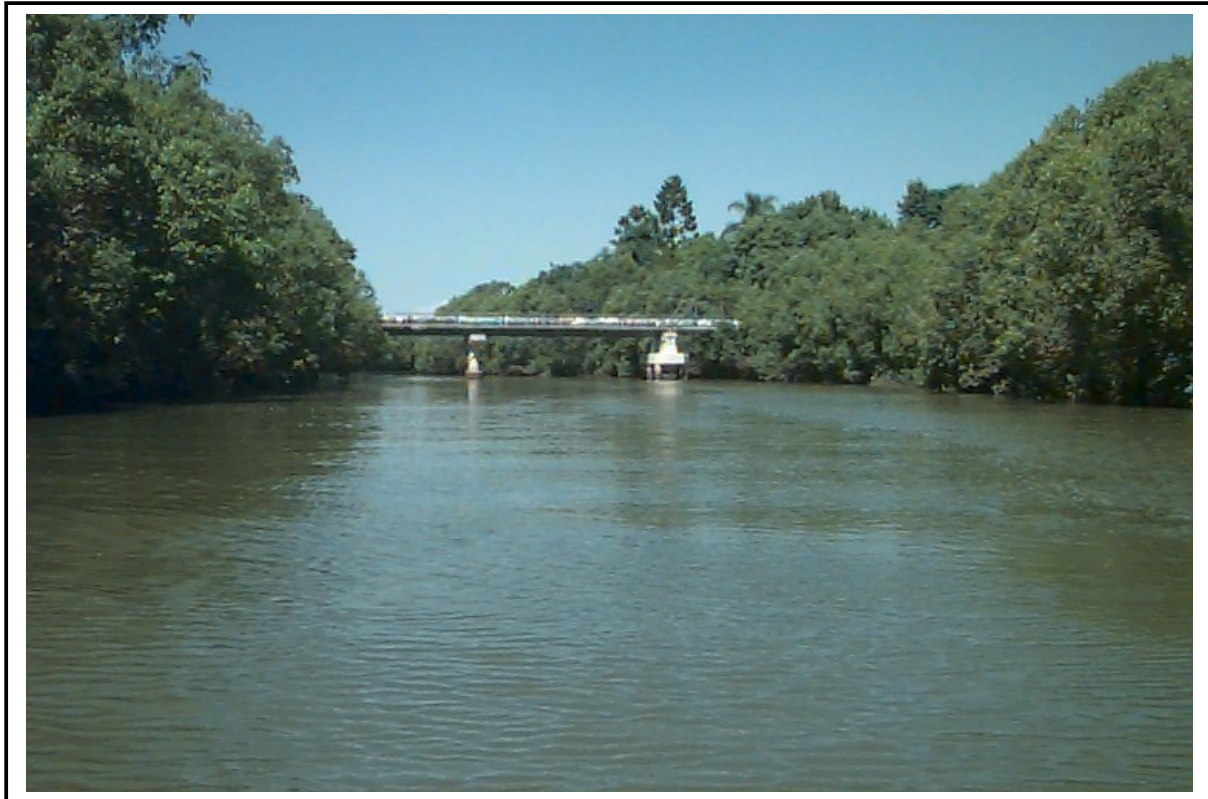
Noble Street Footbridge, looking downstream
