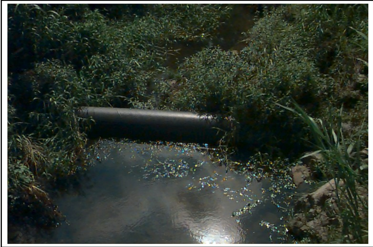
Lugg Street Pipe, looking downstream
