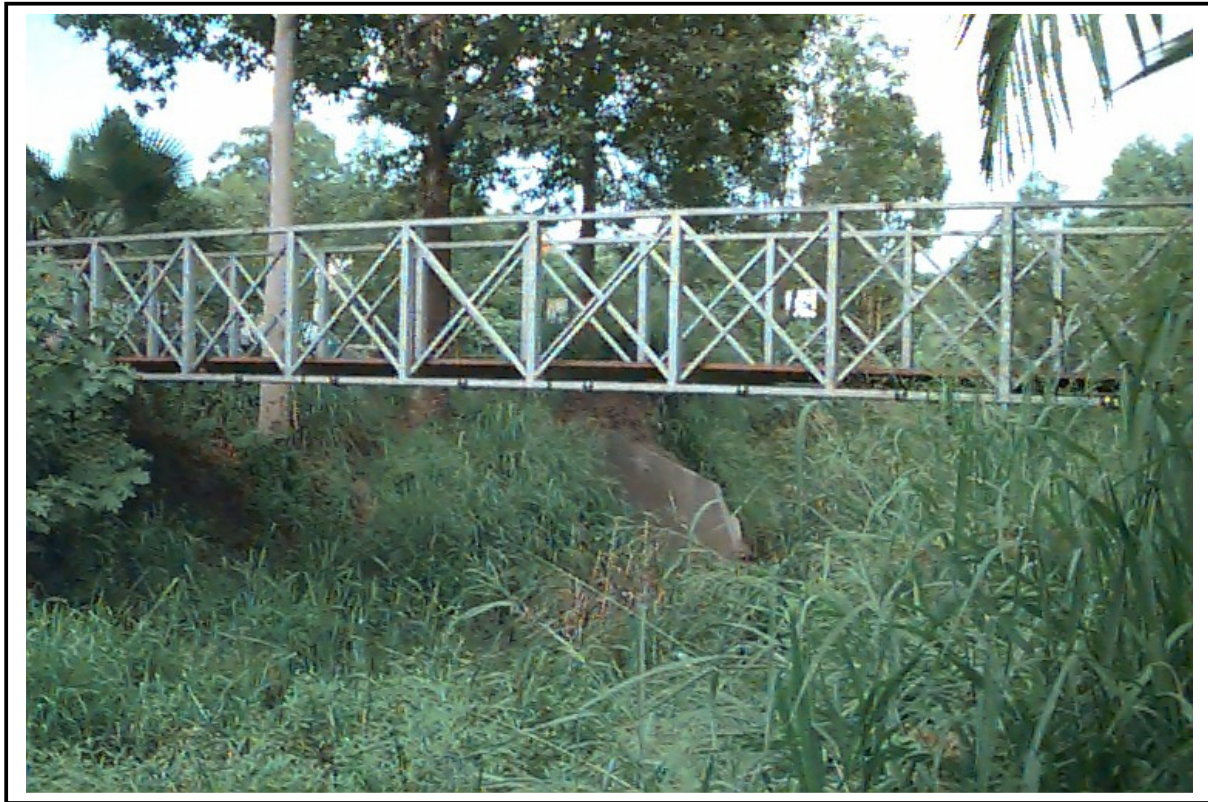
Dean Street Footbridge, looking upstream
