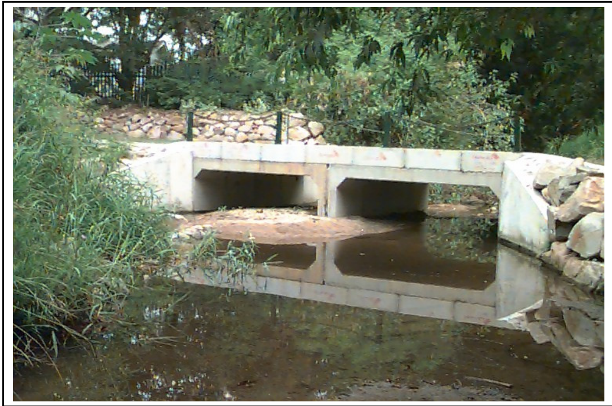
Romea Street, looking upstream
