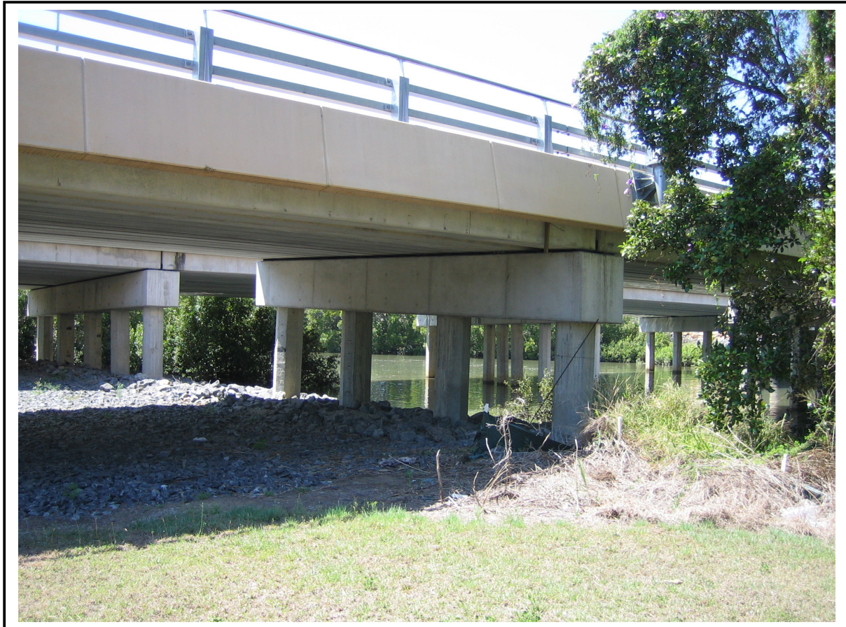
Inner City Bypass Off Ramp (Horace Street), looking downstream
