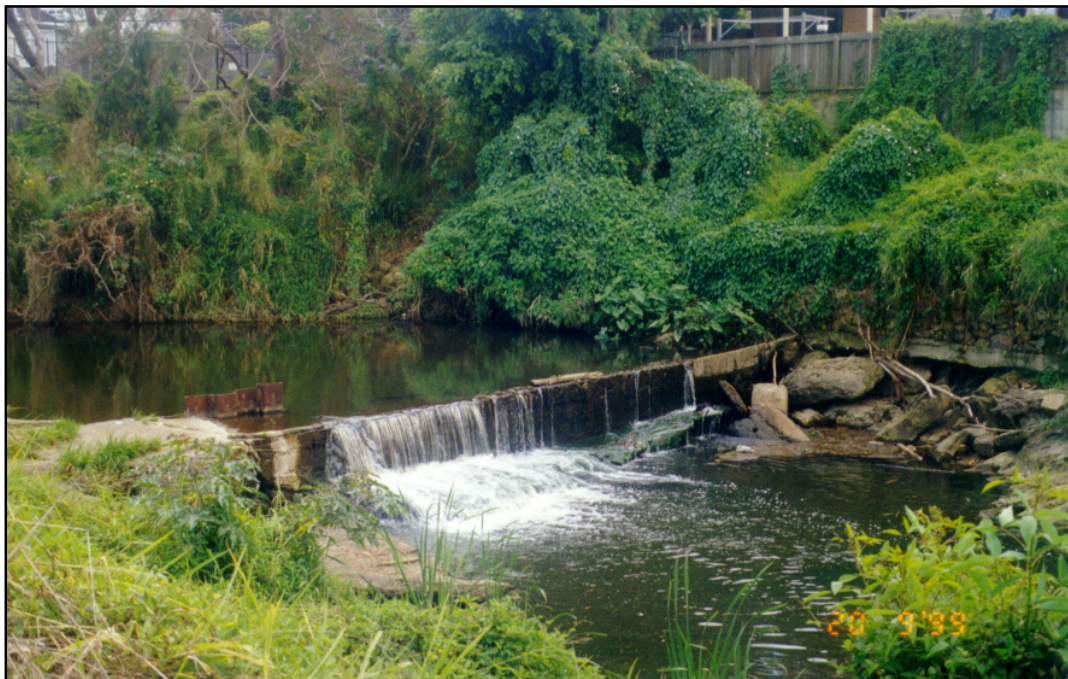
Figure 4.4 Bancroft Park Rating Weir
