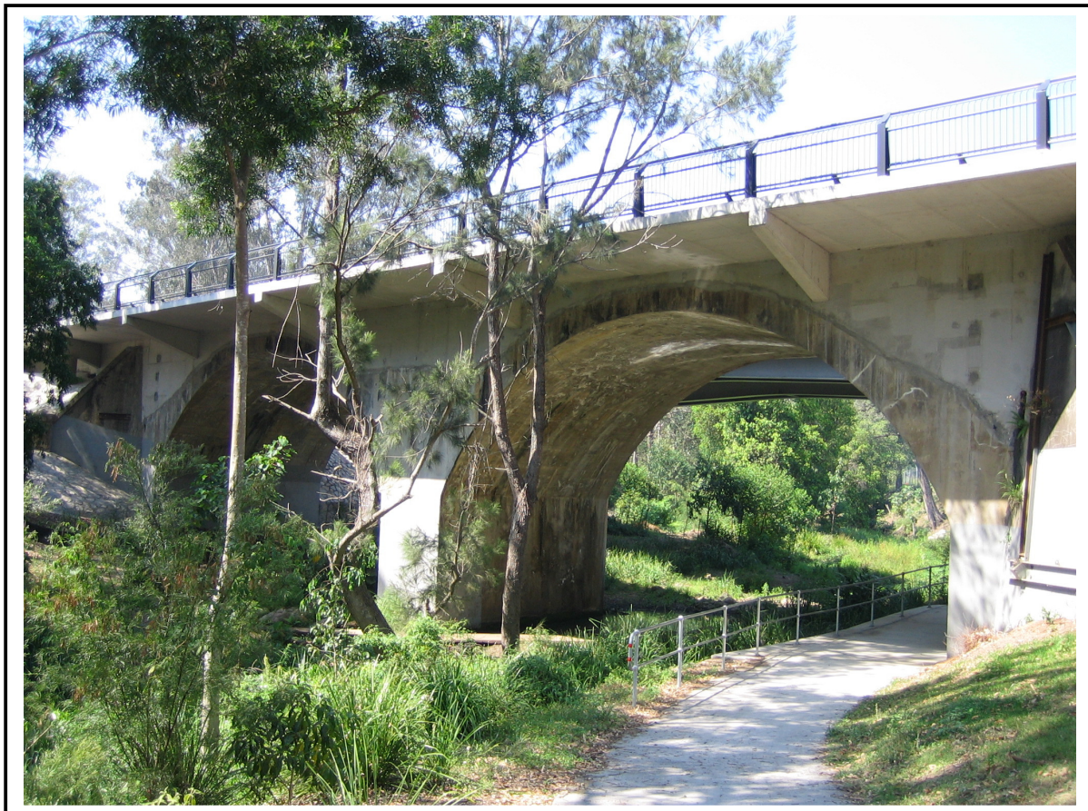
Waterworks Road, looking upstream
