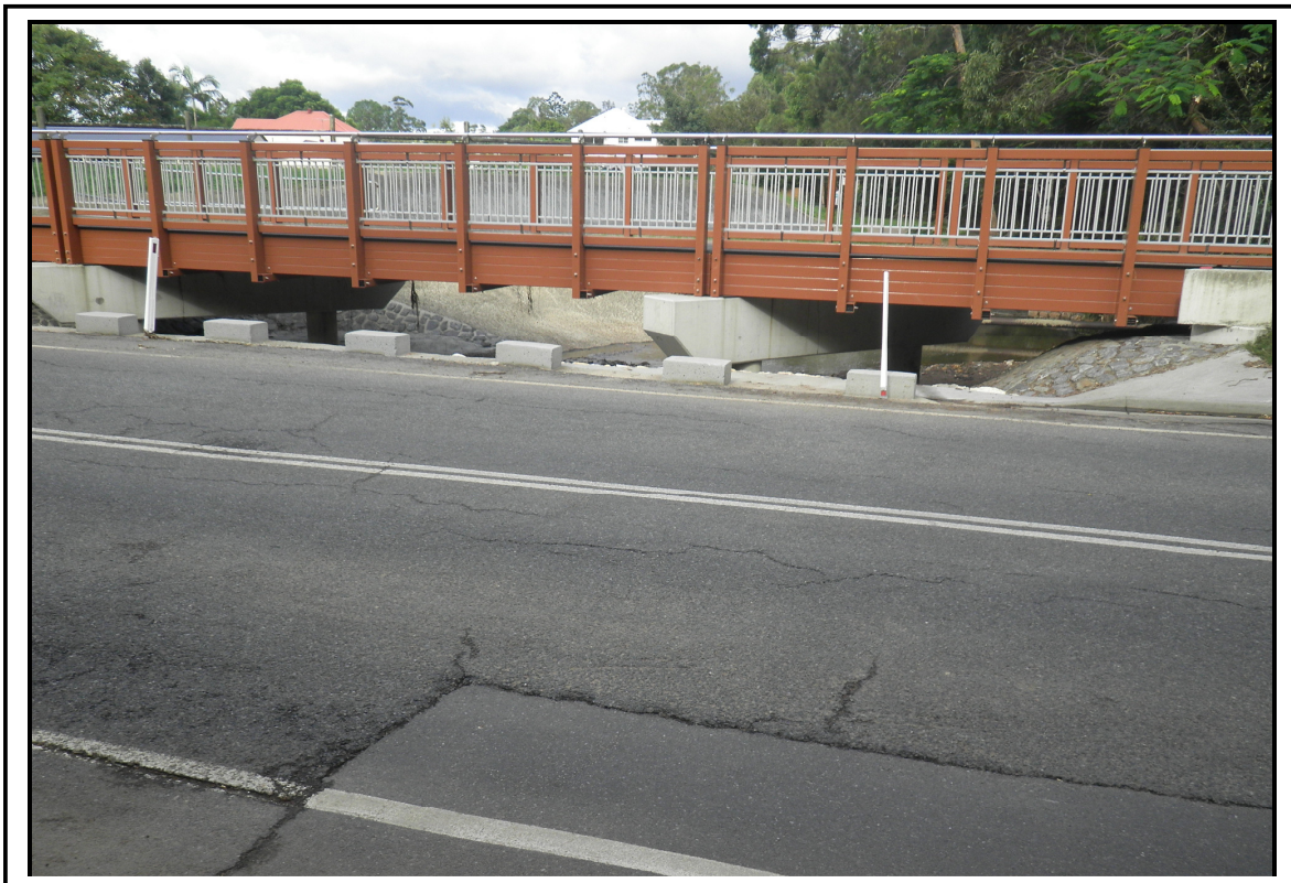
Bowman Parade Footbridge, looking downstream
