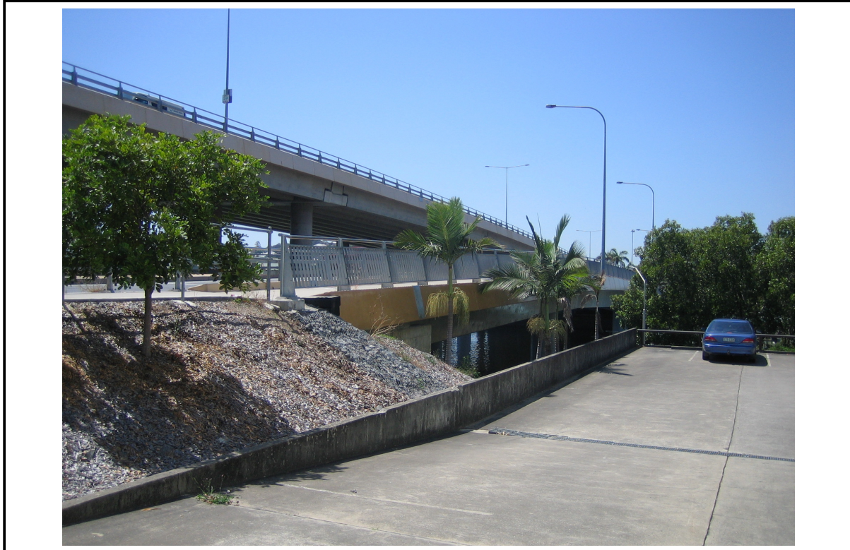
Inner City Bypass, looking upstream (Allison Street in foreground)
